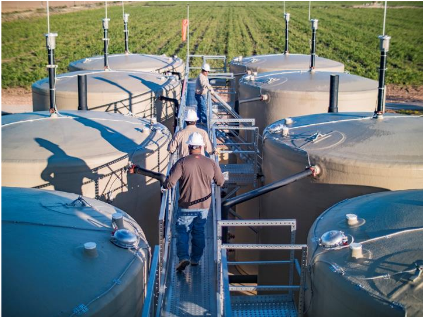
(©Hart Energy, source: Basic Energy Services)
